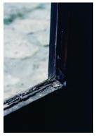
33 years of deep frost developing nightly and washing down the single pane of glass had cause dry rot and after two years empty the glass had slipped into the wood in some places creating air gaps at the tops of the panes.
