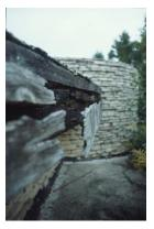
They say a picture says 1000 words. The roof though, technically flat, had a very slight tilt to the rear. There was never anything done to protect the roof's facia from all the runoffs. The water came off the roof to travel over and behind the facia. Of note in this photo is the concrete roof to the shop which has a block wall to the north and the back of the rear kitchen wall to the south. A door from the tunnel connects to this space which is open to the utility portion of the tower.
